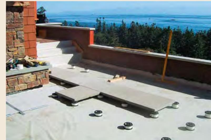
**Level pavers on a sloped deck.** Concrete pavers atop a Duro-Last membrane compose the finished walking surface at the entry court. The pavers are supported at their corners by pedestals that consist of a base, a cap, and a piece of 4-in. plastic sewer pipe ([www.appianway.com](http://www.appianway.com)). Each row of pipes gets a little taller as it moves down the slope so that the pavers end up level. A PVC slip sheet under each pedestal protects the membrane.
